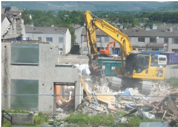
Centre block demolition 2009
