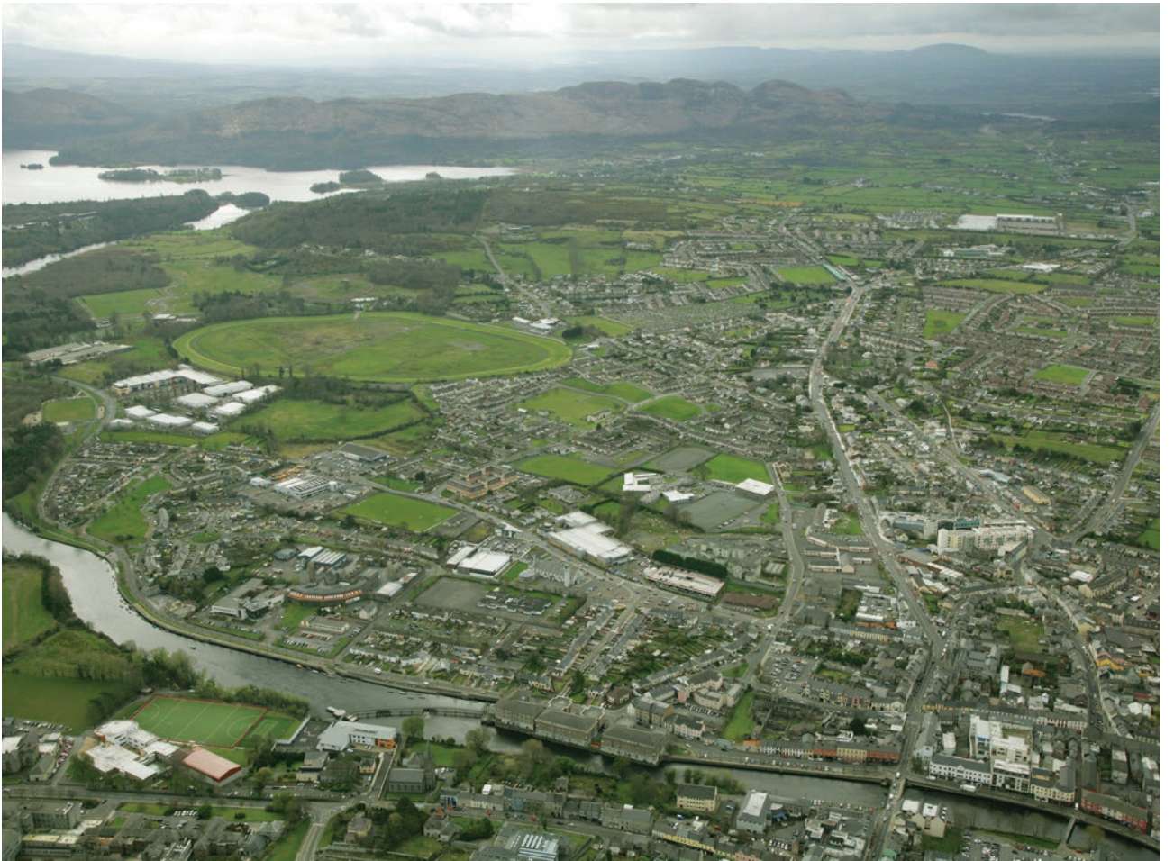
Aerial Photo Looking South over the east city area of Sligo
